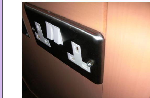
Comments: Loose screw to plug socket
