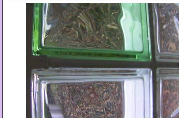
Comments: In-between glass brick grouting.
