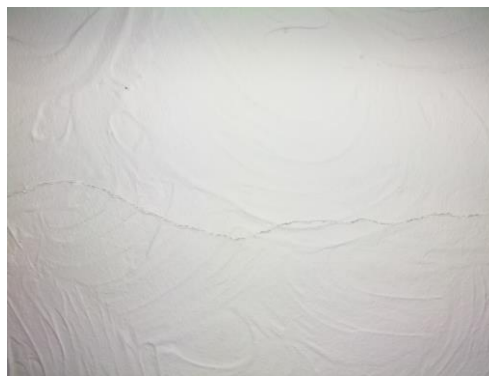
Comments: Hairline crack in ceiling
