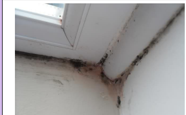
Comments: Mould and mildew on window sills.
